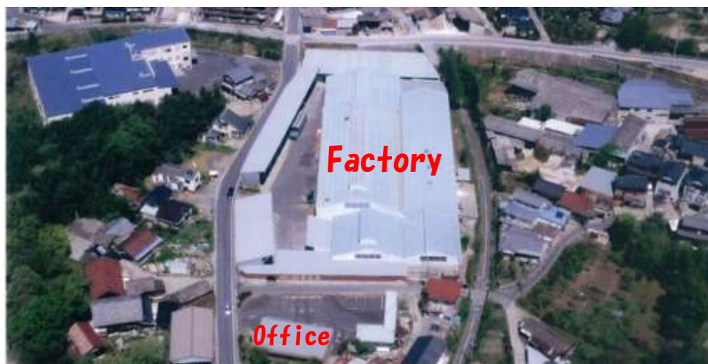
The aerial photo of Gifu Manufactory
