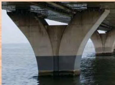
Trans-Tokyo Bay Highway Support Beam
